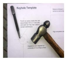
Centre punch hole centres as shown on the template, then drill out the centre pops to 10.5-11.0mm diameter.
